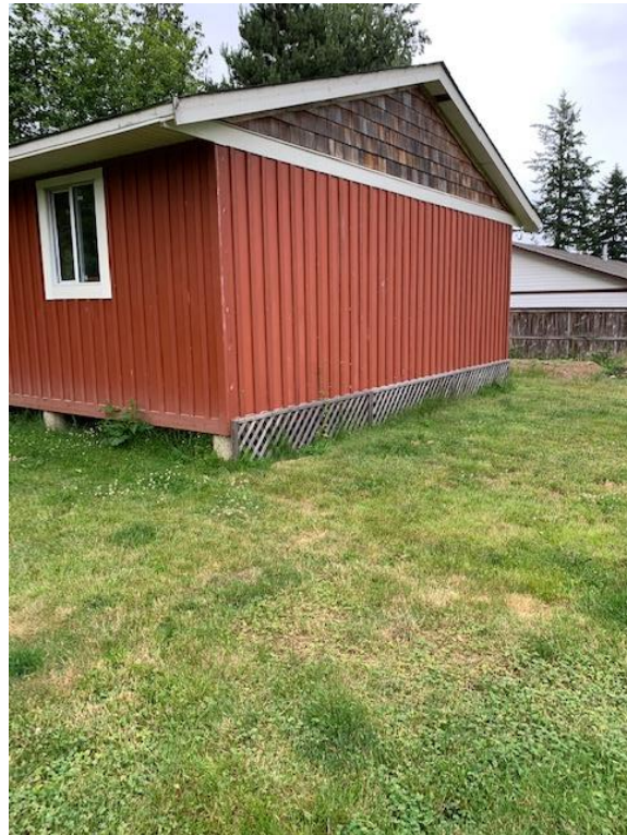
Figure 7: Western Side of Building
