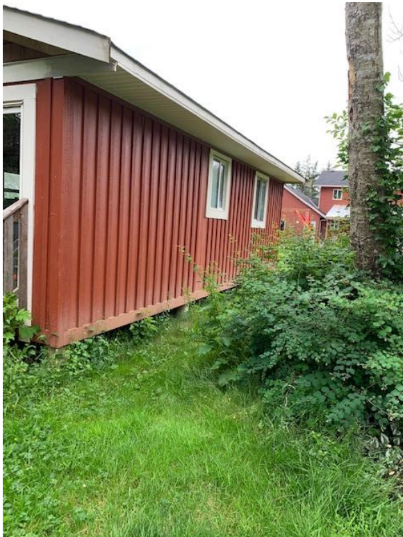
Figure 6: Rear of Accessory Building
